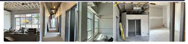
Progress on the new branch is moving along well. Drywall is nearly complete, mudding and taping are underway, and painting has started. Flooring is expected to be installed in July. We're looking forward to seeing the finished space just as much as you are!
