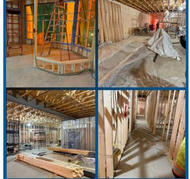
Construction is moving along quickly! Interior walls are framed, windows are going in, and the back brick wall is finished, with other exterior walls underway. Insulation is nearly complete, and the roof should be done by March 21st. Electrical and plumbing are in progress, and drywalling is set to begin in a few weeks.
